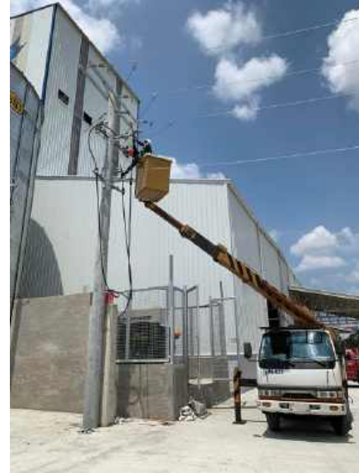
Dan Way - Termination of Power Cable & Transformer Testing
