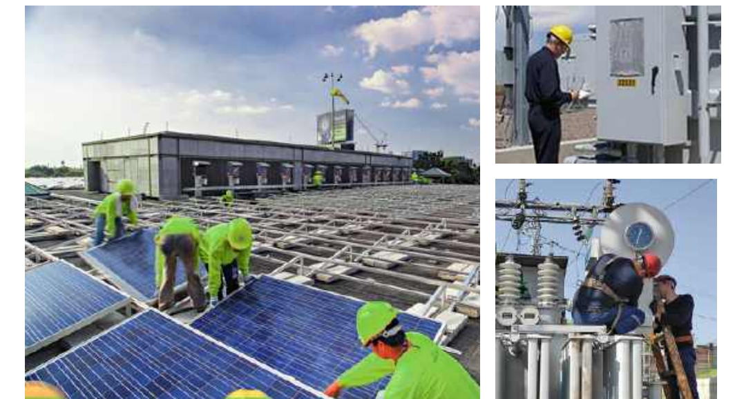
Supply of Potential Transformer –Greenheat Corp.
