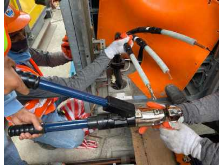
Mindanao Ave. PNR - Termination of Power Cable & Grounding Resistance Test
