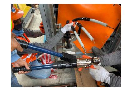
Mindanao Ave. PNR -Termination of Power Cable & Grounding Resistance Test
